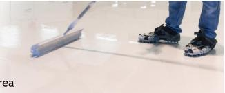
Polymères liquides innovants à hautes performances Innovative high-performance liquid polymers Solvent based polyaspartic polyurea coating system, Low Solids
